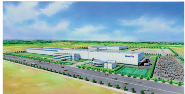
Image of the Ibaraki Plant upon completion
